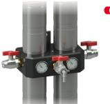
6 By opening the stopcock on the water outlet side, the home supply is put into operation. The water outlet side is marked by a label. In order to remove already existing contaminations from the piping system, the water should flow for approx. 2-3 minutes from each tap in the house after the QUADRO installation has been completed. It is advantageous to clean all the aerators in the house in order to wash out the coarsest dirt.
